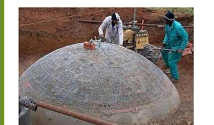
Medium scale anaerobic digesters available (Fixed dome and flexible balloon-type) installed by Green Heat, Uganda.
